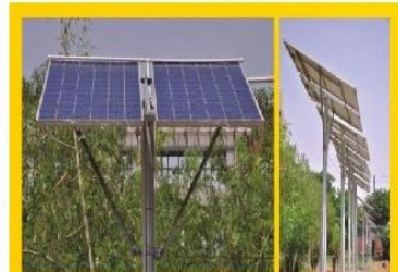
Dust Cleaning on Solar Panels using water from Solar Water Pump
